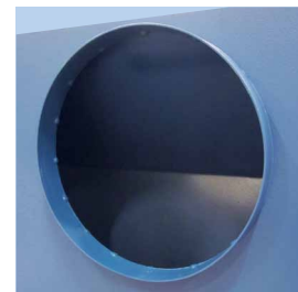
Inlet Placed in the top left side, after which the air is turned down.
